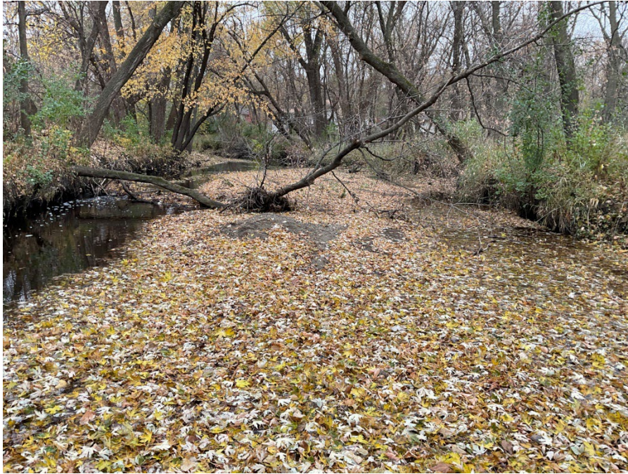
Photo 31: Site 3c. Undercut at the upstream section at station 46+50.
