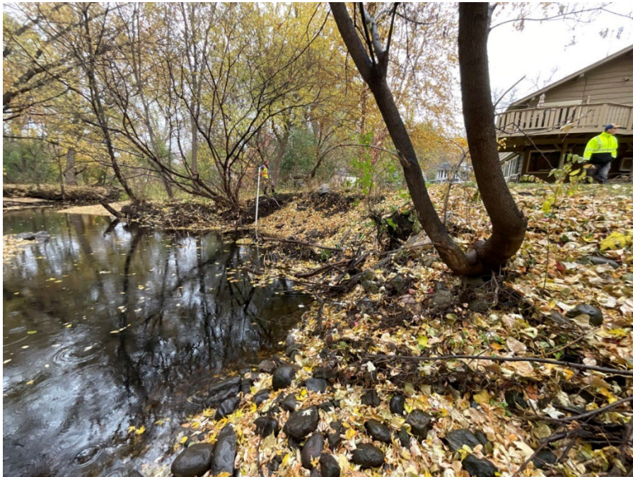
Photo 26: Site 2m. Soil exposure and deposition at the right bank of station 35+60 (facing downstream).
