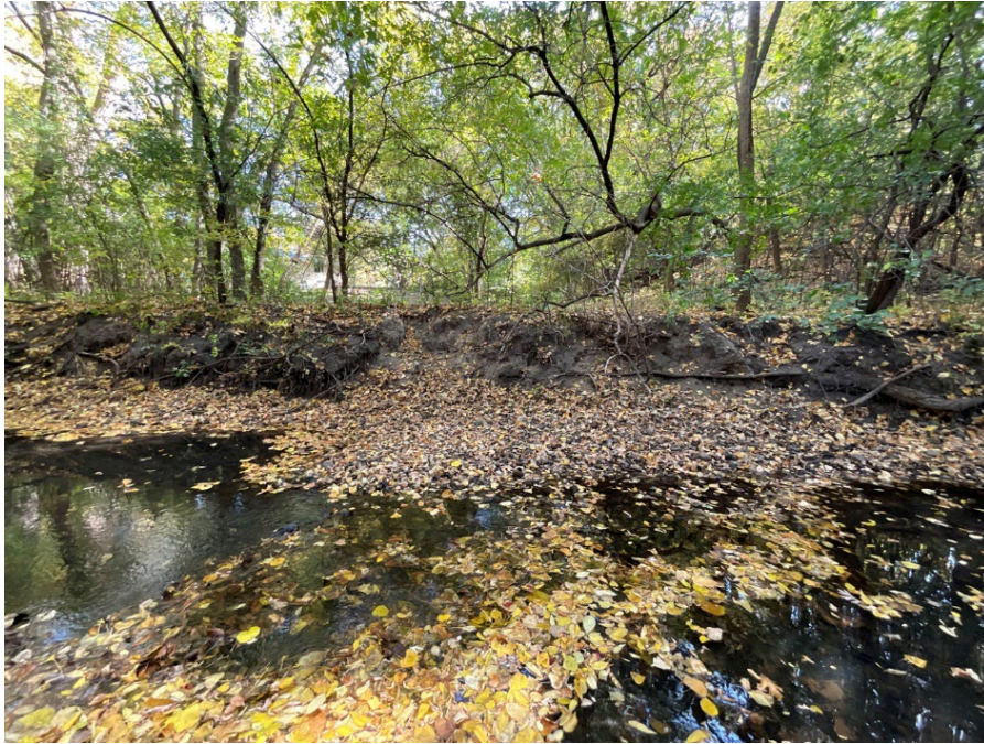
Photo 9: Site 1f. Bare soil at the right bank of station 12+30.
