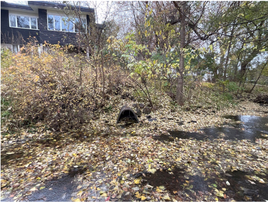
Photo 23: Site 2j. Left bank outlet at station 31+00 directly upstream of a sanitary sewer that crosses the creek.
