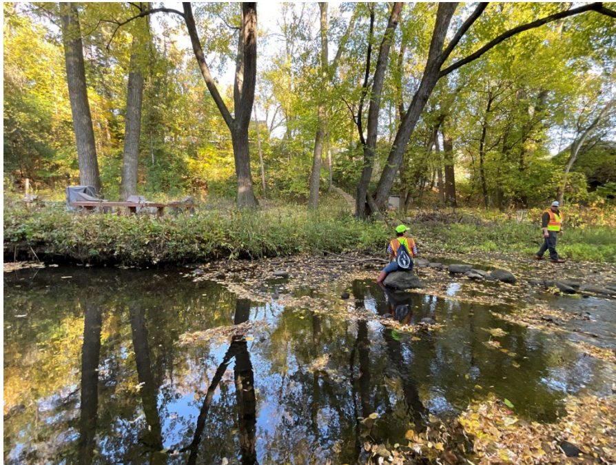
Photo 18: Site 2f. Left bank undercutting at station 23+10.
