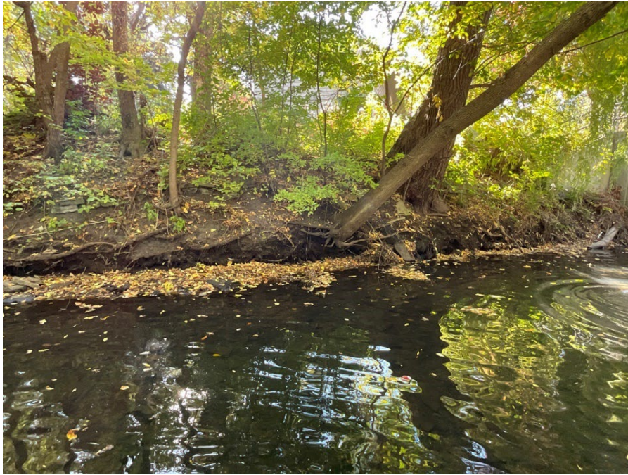
Photo 1: Site 1a. Bare soil on the right bank at station 0+40.
