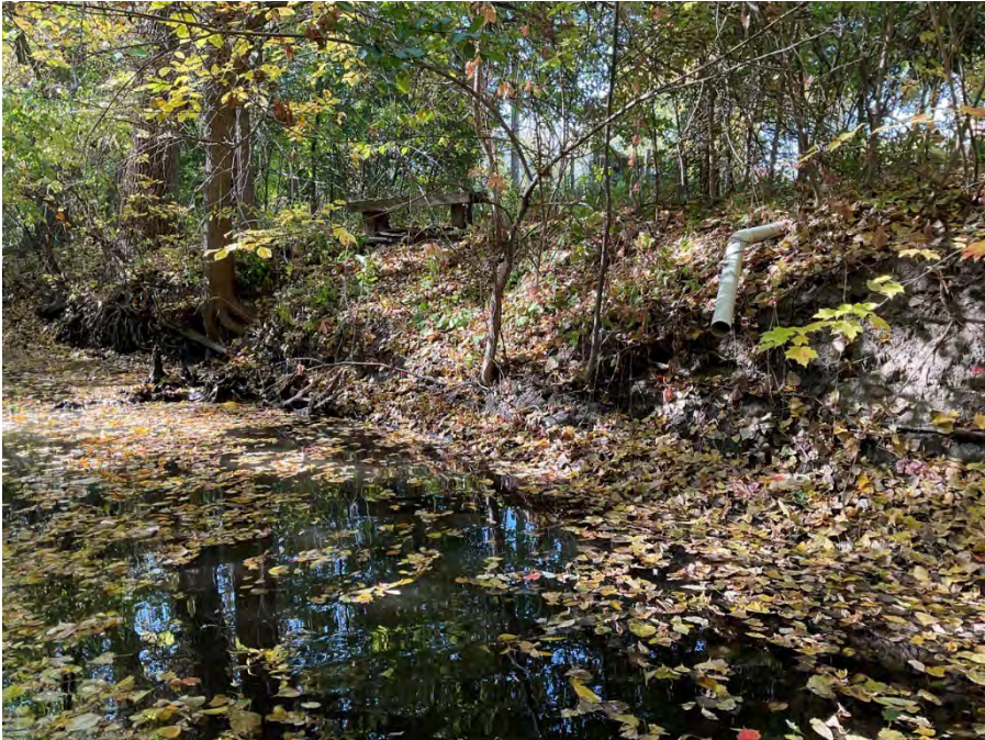
Photo 8: Site 1e. Drainpipe and bare soil on the left bank of station 13+50 (facing upstream).
