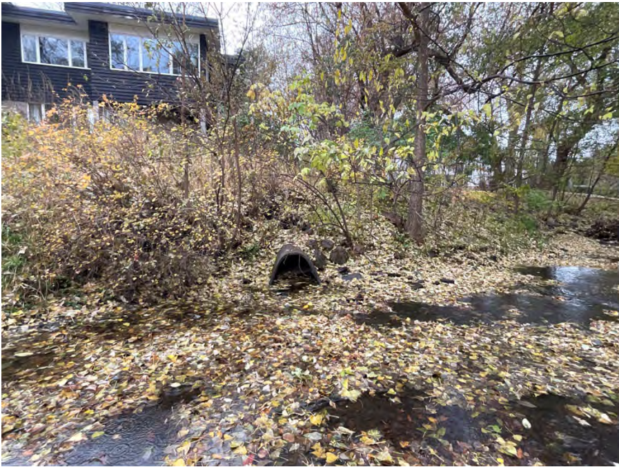
Photo 23: Site 2j. Left bank outlet at station 31+00 directly upstream of a sanitary sewer that crosses the creek.
