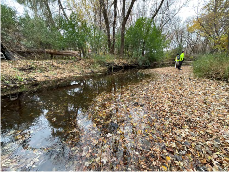
Photo 30: Site 3b. Undercut on the left bank of station 42+70. Deposition on the right bank (facing downstream).
