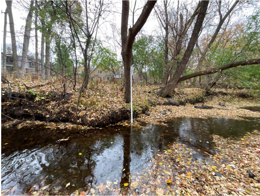
Photo 25: Site 2l. BEHI measurement and undercut at the left bank of station 34+25.
