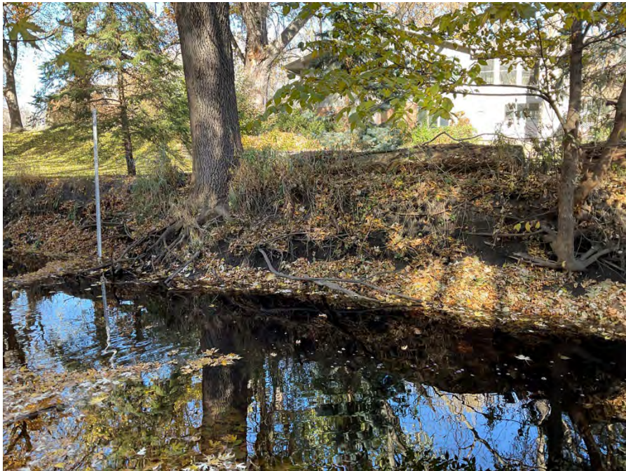
Photo 34: Site 3f. Bare soil at the upstream section at station 50+90.
