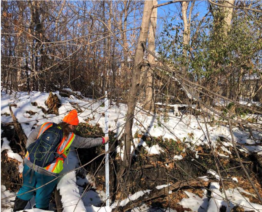
Figure 3-3 Left Bank Erosion (Reach 1)
