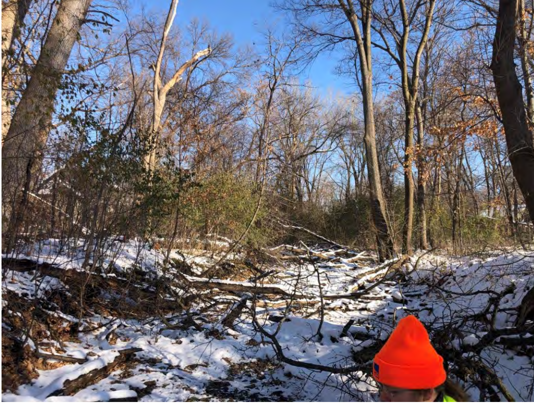
Figure A- 7 In-channel debris leading to bank erosion and sediment aggradation.
