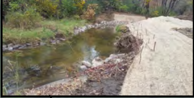
Example Rock Toe (Left) and Coir Blanket/Live Stakes (Right)
