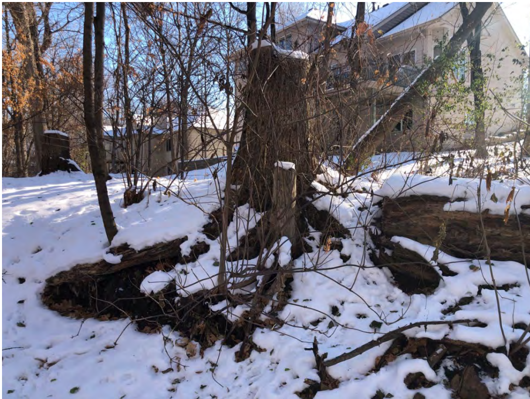
Figure A- 2 Right bank erosion.
