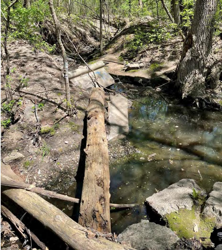
Figure 5-6 Pond SR-4 Downstream Outlet Channel Erosion and Construction Debris
