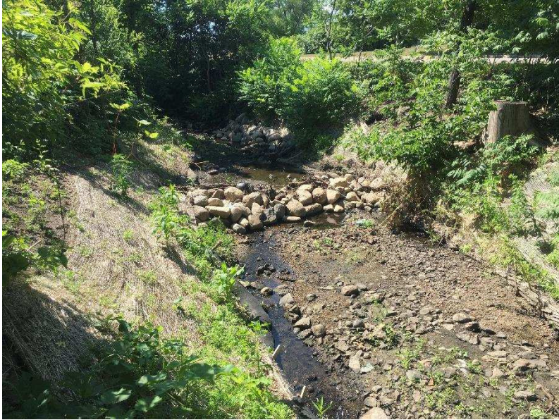
After construction: August 2022
