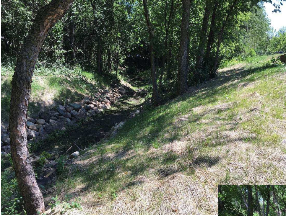
After construction: August 2022
