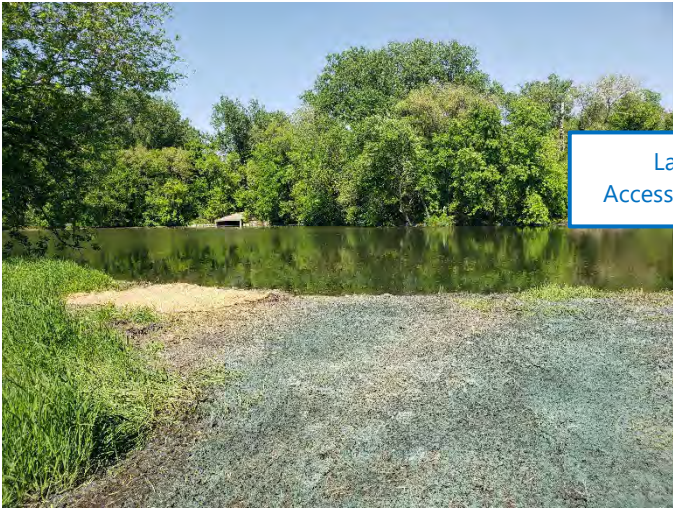
Lagoon D Access Restoration
