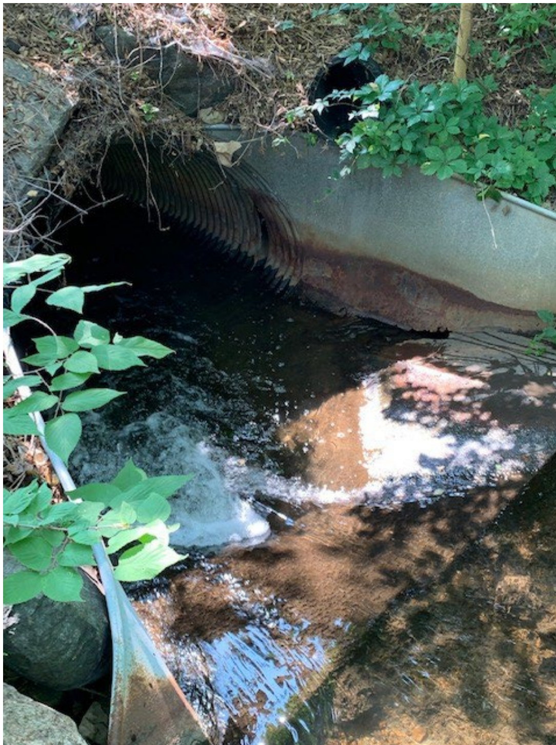
West end of culvert (inlet)
