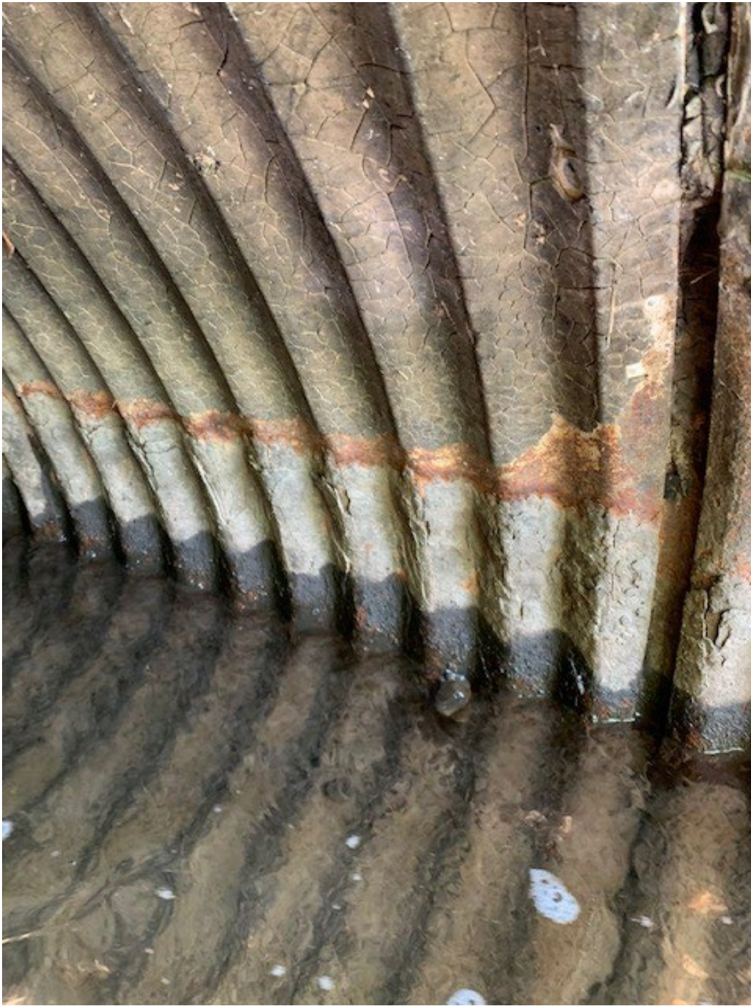
Inside of culvert
