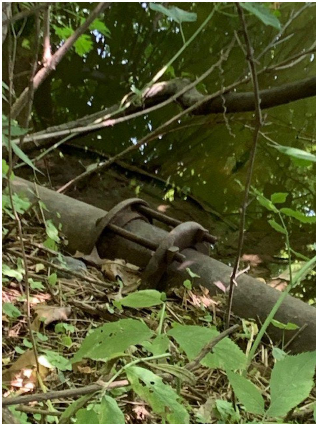
East end of culvert (outlet) – under water. Unknown pipe in foreground
