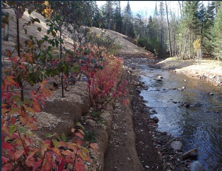
Vegetated Reinforced Soil Slopes
