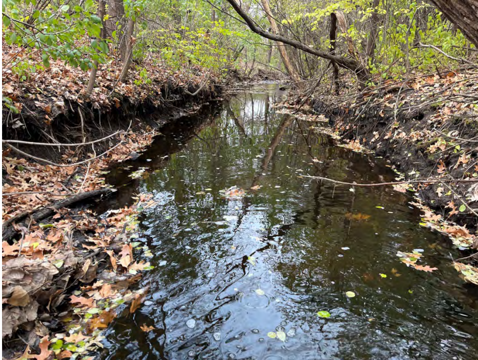
Photo 36: Site 4c. Looking downstream at station 60+00, the left bank is undercut.
