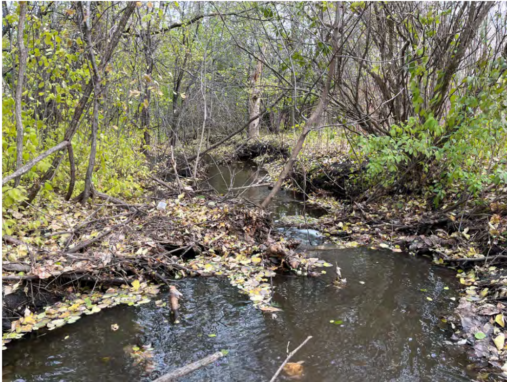
Photo 12: Site 1g. Looking downstream at station 15+10, multiple outlets enter this location and could contribute to the eroding banks.
