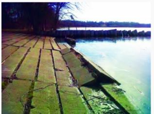
The concrete planks that comprise the French boat launch on Medicine Lake frequently fail and require sufficient maintenance. Per scheduled improvements, Three Rivers will reconstruct the ramp beginning after Labor Day 2014. (Courtesy of Three Rivers Park District)
