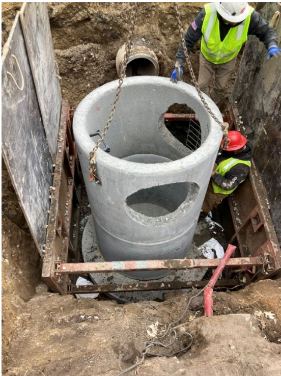
Construction of sump manhole
