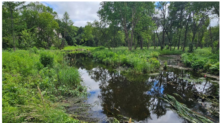
Post construction after significant rain
